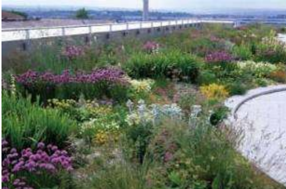
Moorgate Crofts Business Centre, a “business incubation centre” featuring geothermal heating and cooling, and a conference centre emerging from a green roof (RMBC)
